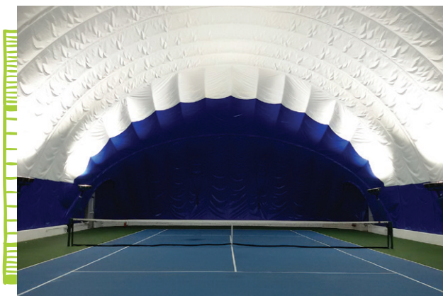
Tennis bubble was replaced with one of better thermo-insulating effect, reducing 35% of energy consumption compared to 2014 (Pacific Club)
