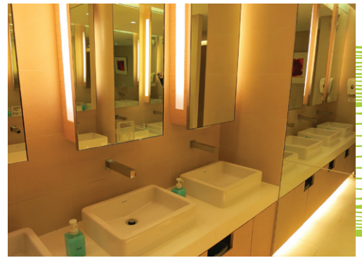
Replacing conventional toilet basin tap with automatic sensor faucets, saving about 25% of water usage (Pacific Club)
